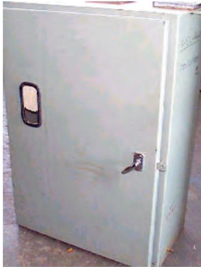
Fig. 17.3: Mechanism box with local control unit
