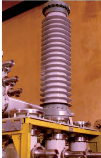
Fig. 5.16: Gas-to-air termination with composite insulator housing
